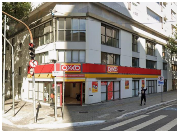
FACHADA DO CONDOMÍNIO (VIA GOOGLE STREET VIEW)
